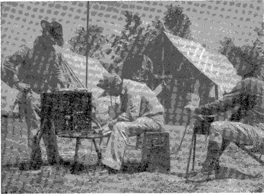
Portable field transmitter-receiver in operation. Soldier at right turns crank of a hand generator, used to charge batteries supplying current to the set. Courtesy U. S. Signal Corps.
